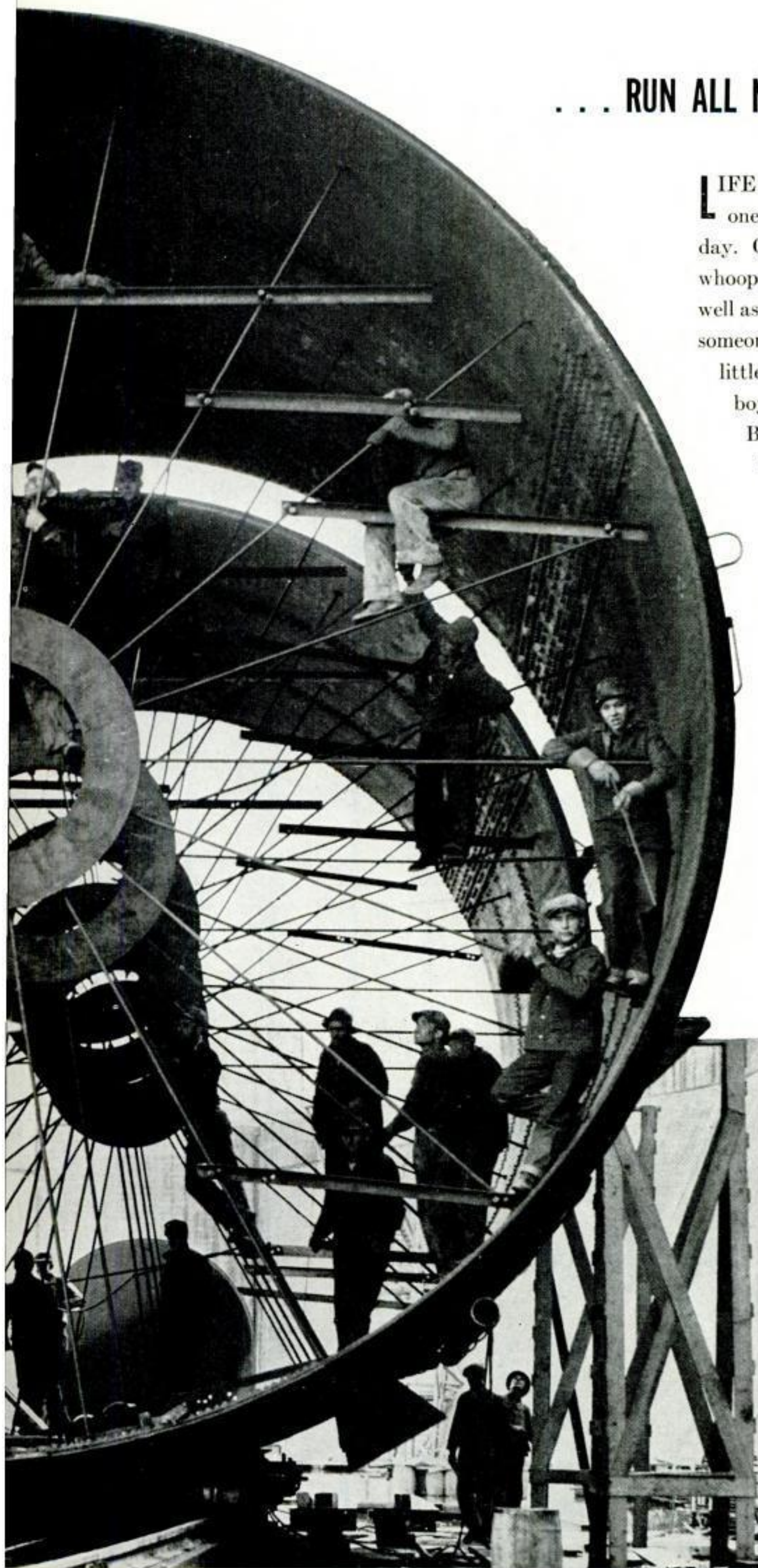
ILL RUN THROUGH THIS STEEL "LINER"
