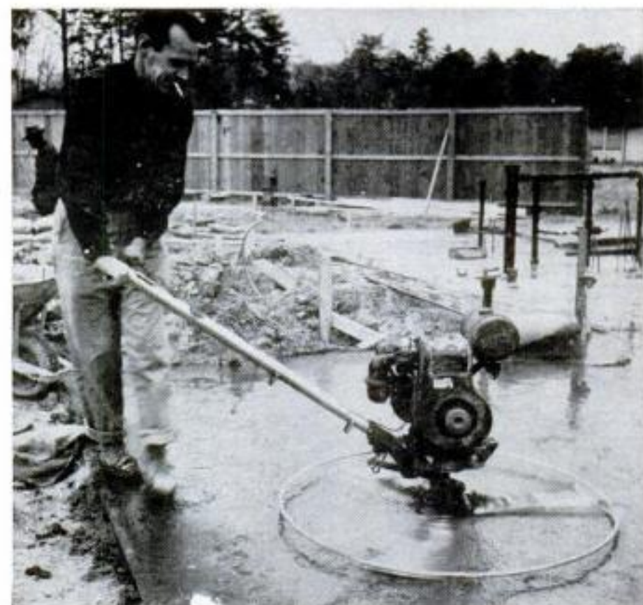
SHREVEPORT, LA. Workman is smoothing terrazzo with mechanical trowel. Use of terrazzo gives entire house uniform, unbroken, durable flooring—easy to put in and to keep clean. (Builder: Frank Zuzak)
