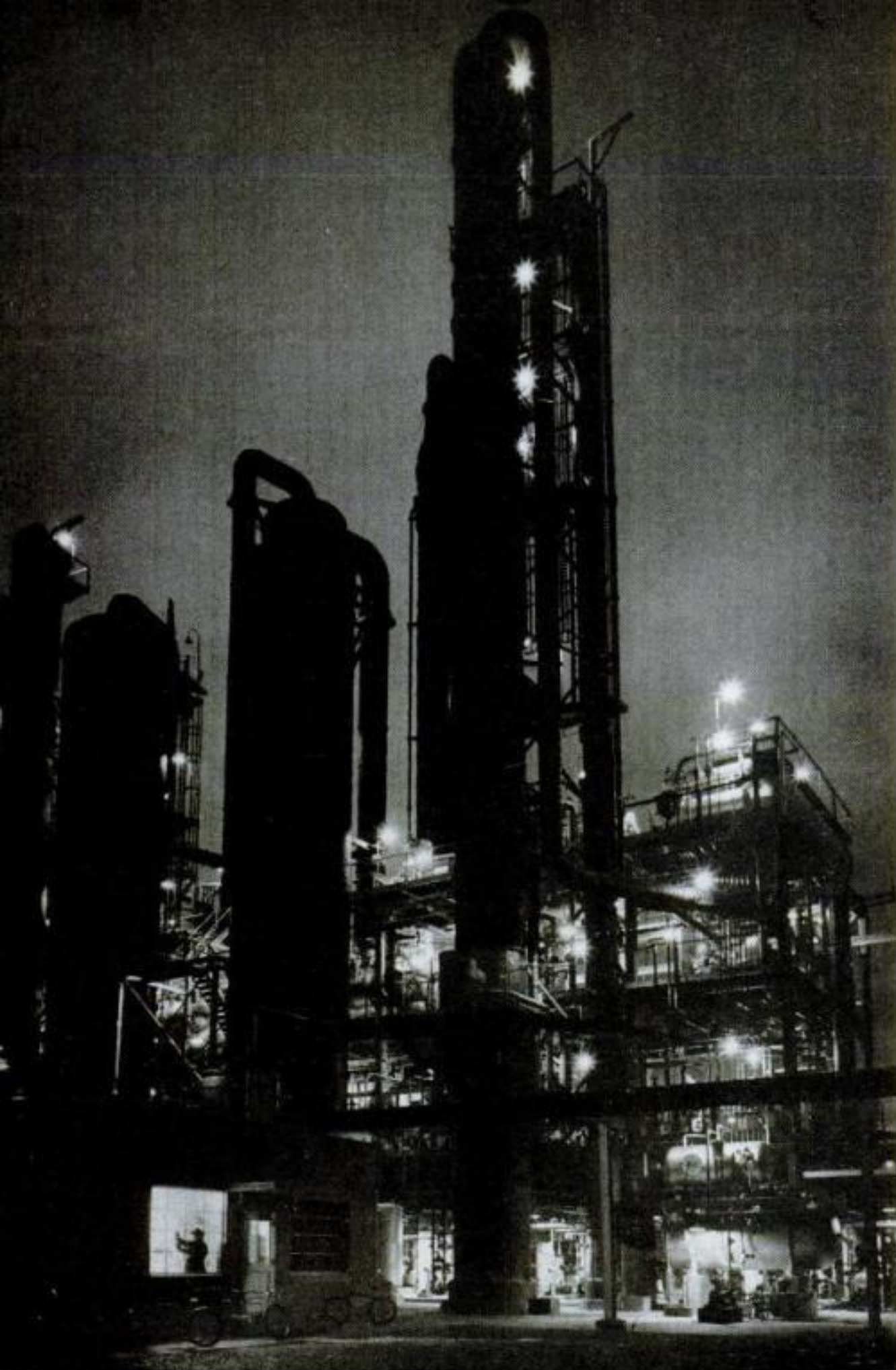
RISING TOWERS of Texas City plant on Gulf Coast make styrene, used in rubber, paint, plastics. Silhouetted chemist tests samples in control room.
