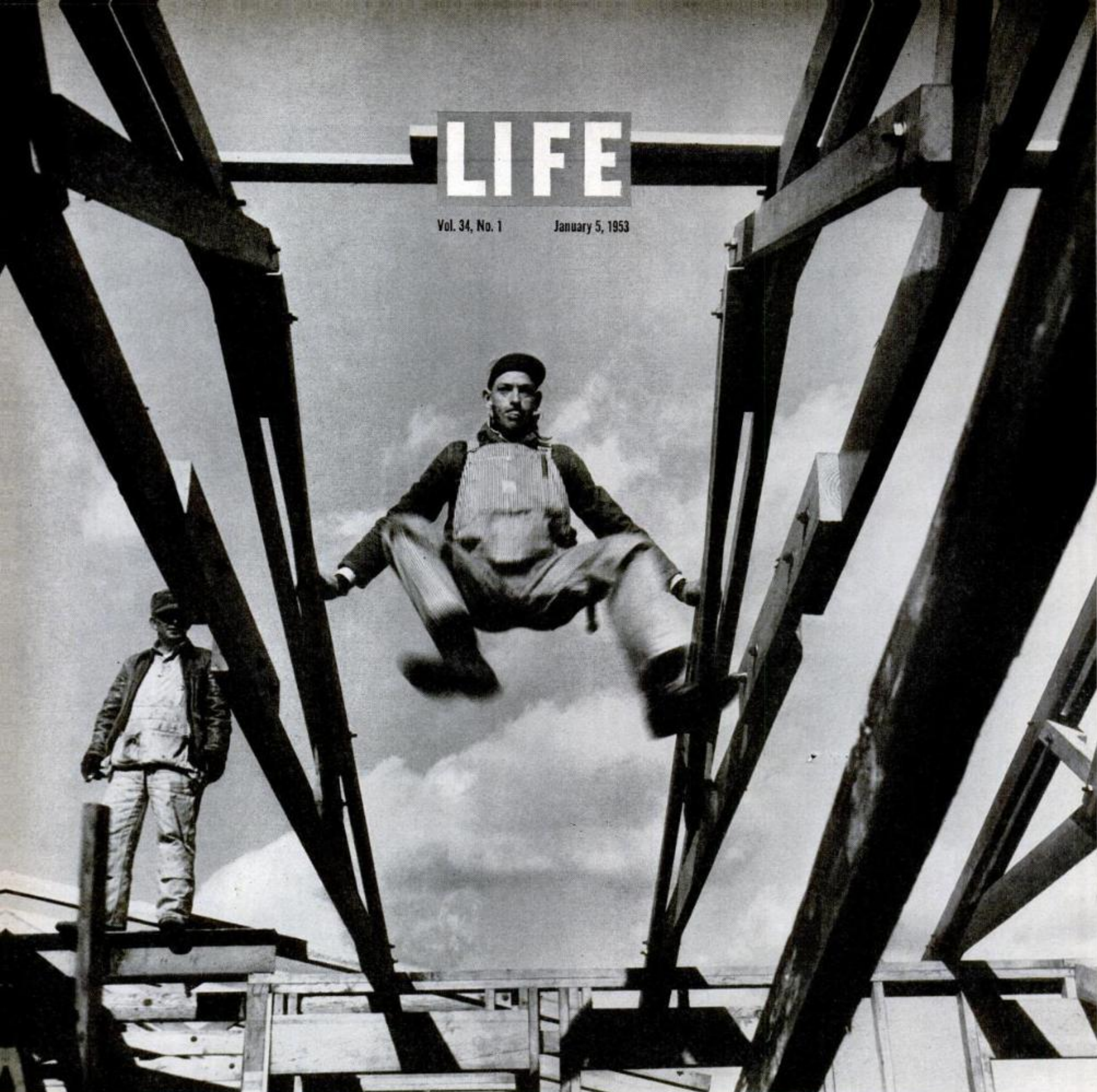
IN MIDWEST CITY, OKLA., W. P. ATKINSON HOUSE, WORKMAN SWINGS HIMSELF TO CENTER OF PRECUT, PREBOLTED ROOF TRUSSES TO NAIL PEAK IN PLACE
