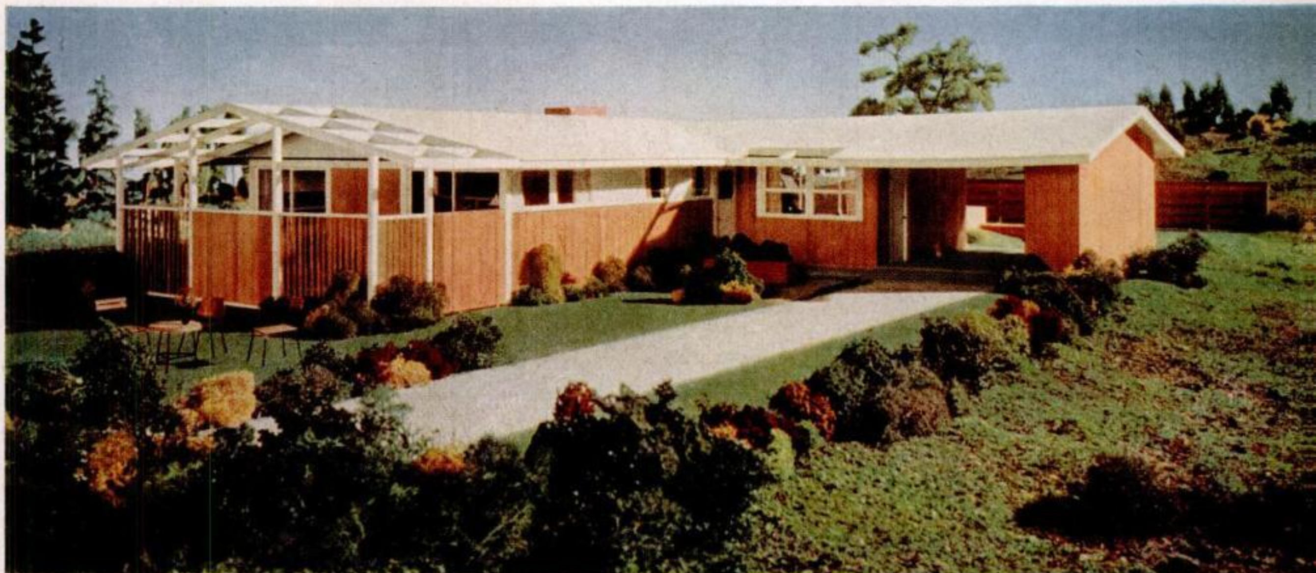
ENTRANCE VIEW shows side of house facing street. Siding is redwood; roof is white marble chips. Roof overhang makes sheltered path to front door, which opens on entrance hall. Family entrance leads from carport to kitchen; just
