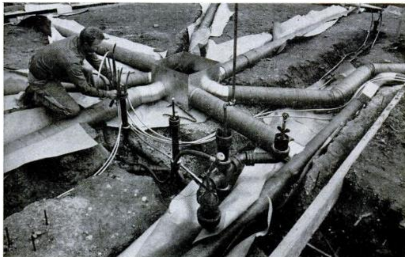
DAYTON, OHIO Simplest way to install water pipes, waste pipes and heating pipes that can carry air conditioning (large ones above) is to arrange them on
