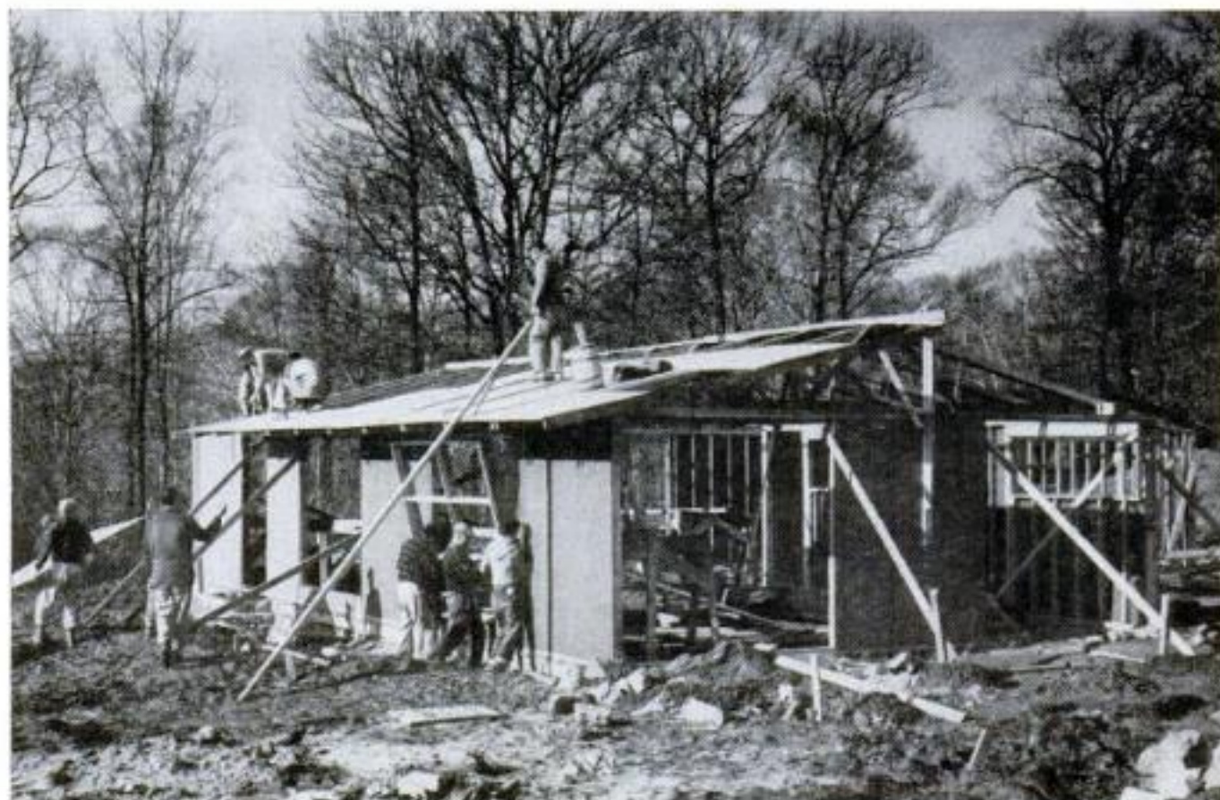
LIMA, PA. Workmen swarm over house. They are setting in windows, tossing up and nailing down roof sheathing, all simultaneously. With so many pre-cut and
