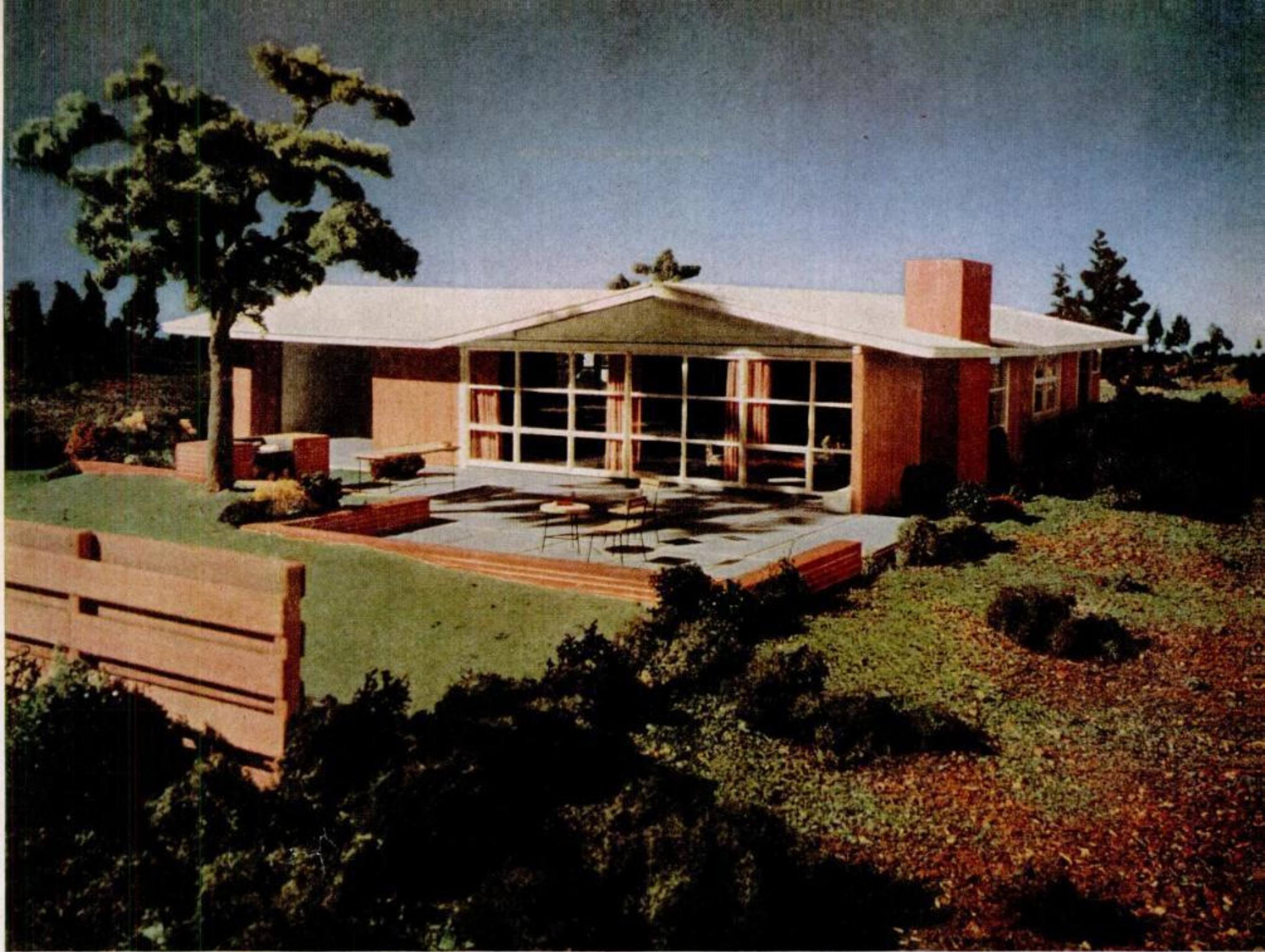
MAIN LIVING SECTIONS of the house, behind a bank of windows, face away from the street onto a terrace and backyard which is screened by a redwood fence. Two sections of the window slide open to provide access to terrace. Red
