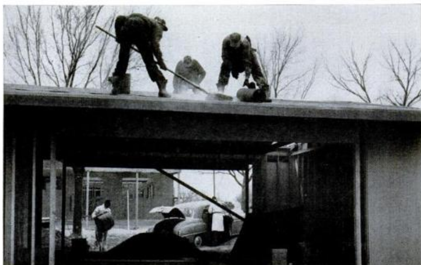
WICHITA, KANS. After roof trusses are quickly lifted and secured in place, plywood is spread over them. Above: workmen are shown putting
