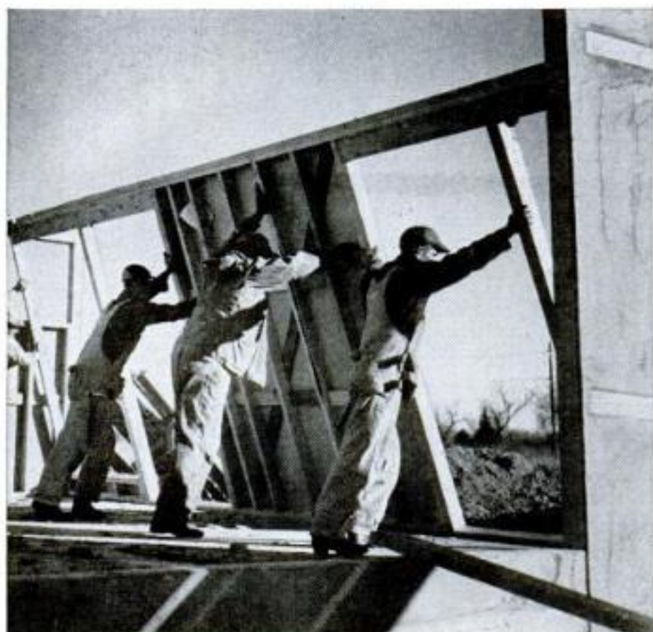
DENVER, COLO. Workmen tilt wall into place. Sections are assembled on "deck" of house before they are pushed up. Windows slip into exact place in walls so that no extra fitting is needed above them. (Builder: Franklin Burns)
