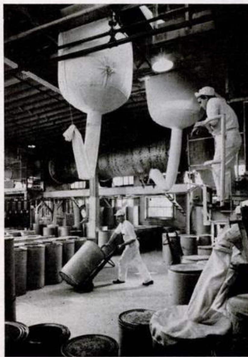
WORLD'S BIGGEST SINGLE CHLORINE PLANT IS OPERATED BY MONSANTO FOR U.S. AT MUSCLE SHOALS, ALA. ELECTRODES EXTRACT CHLORINE FROM BRINE
