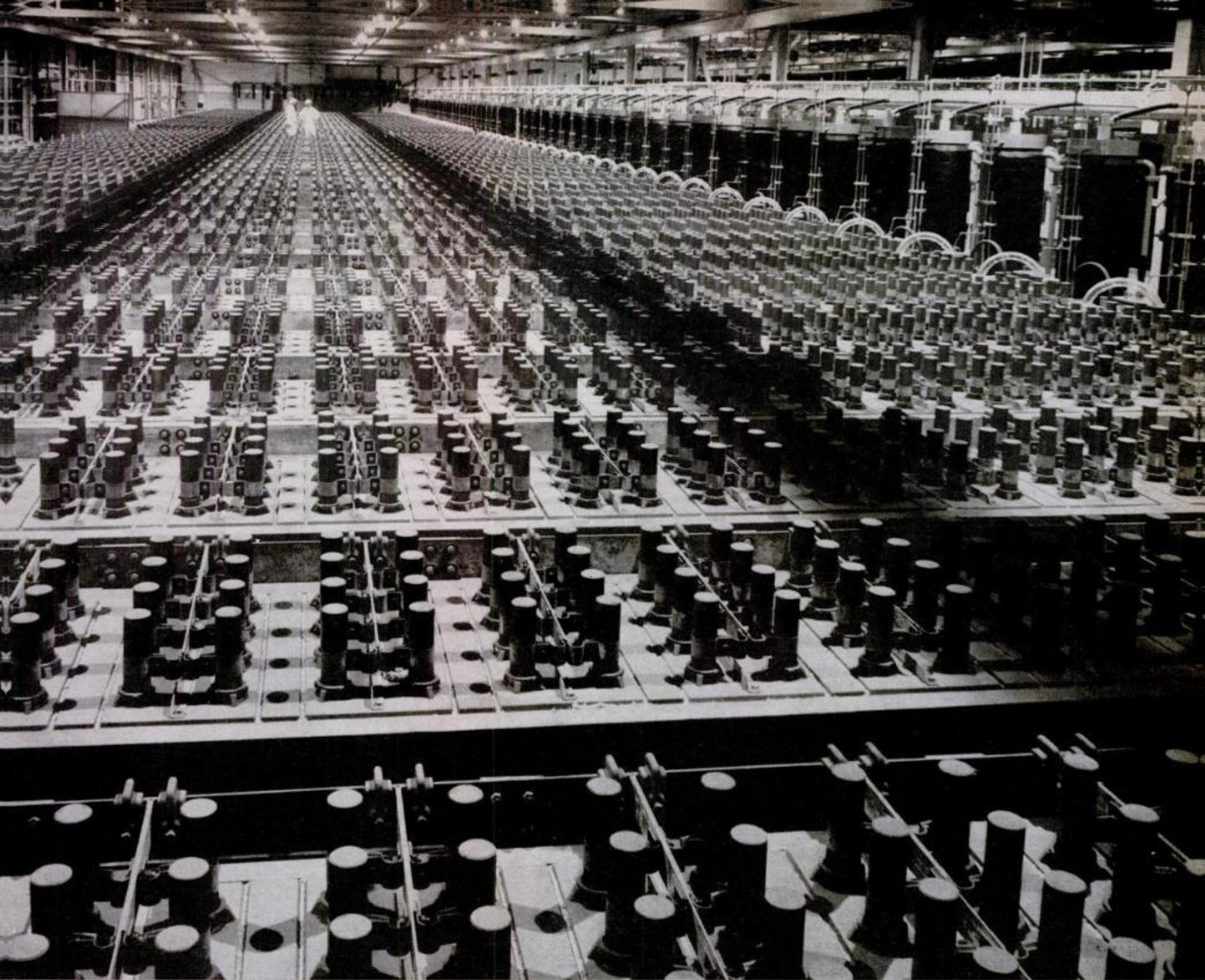
WORLD'S BIGGEST SINGLE CHLORINE PLANT IS OPERATED BY MONSANTO FOR U.S. AT MUSCLE SHOALS, ALA. ELECTRODES EXTRACT CHLORINE FROM BRINE
